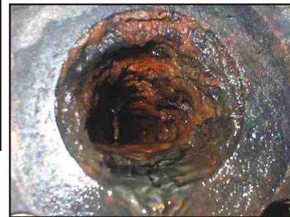
November 03, 2006 After installation
