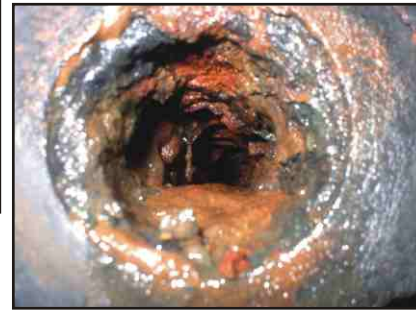
August 11, 2006 After installation
